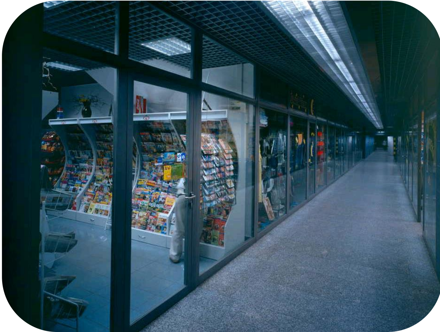
Tube station, Warsaw 15 mm Pilkington Pyrostop ® 30-10
